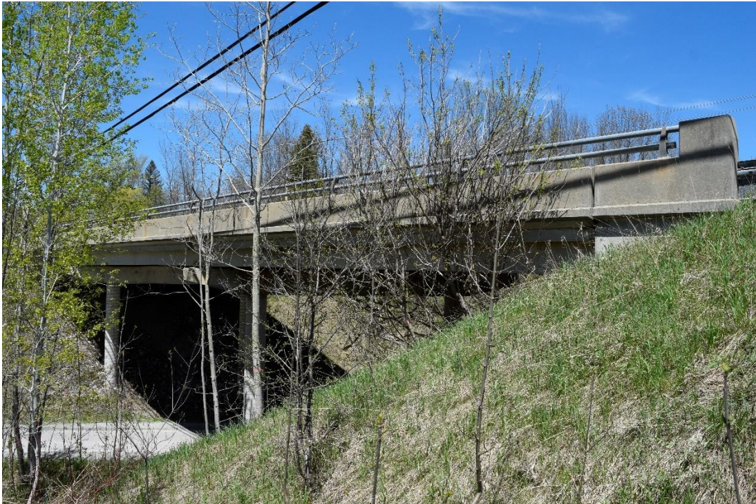
Image 1: Overview of Old Fort Road Overhead Bridge, facing southeast
