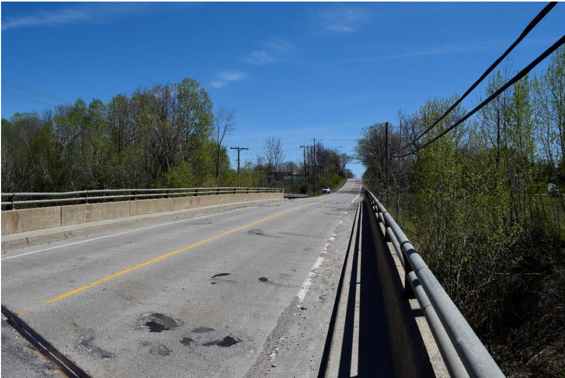
Image 6: Surface of bridge deck, facing west
