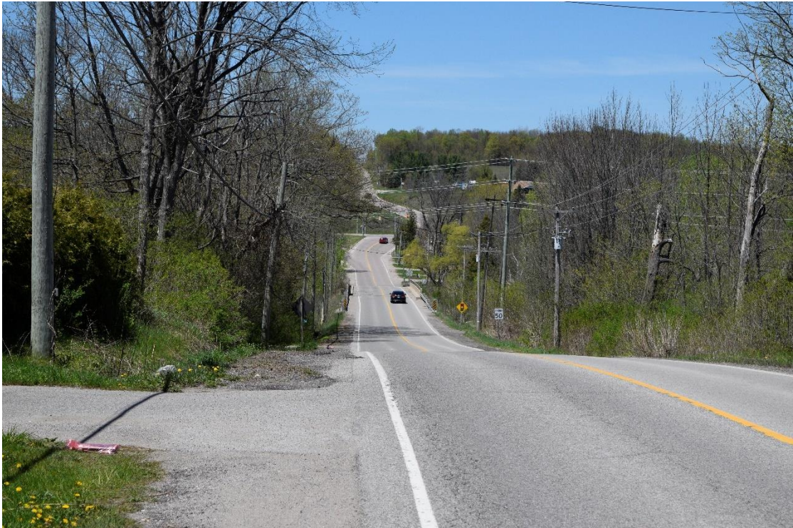
Image 2: West approach to bridge, facing east
