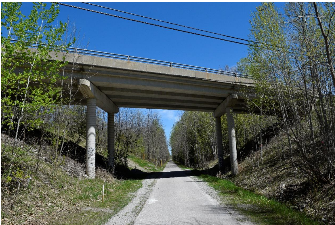
Image 4: Bridge as viewed from Tans Canada Trail, facing south
