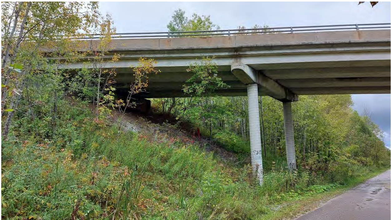
Photo 2: South bridge abutment/embankment, from the TransCanada trail, facing west.
