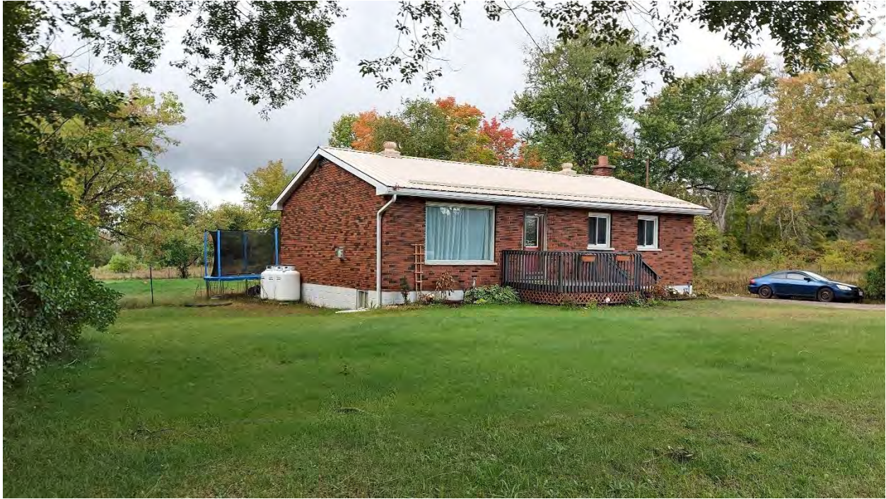
Photo 5: 2852 Old Fort Road residential home, propane heating tanks typical of the houses in the APU Study Area are visible.
