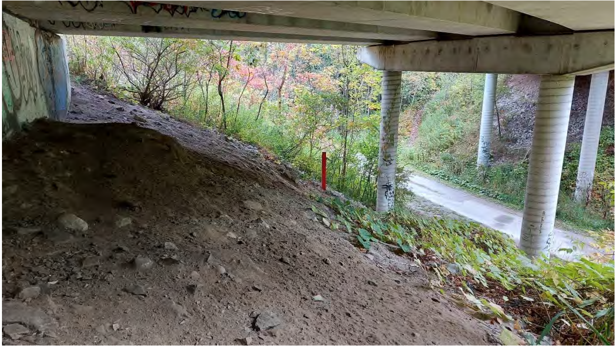
Photo 3: Underside of the bridge, view of the north embankment, facing southeast.
