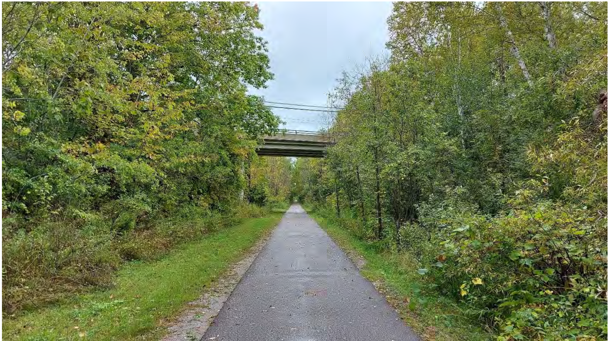
Photo 4: View of the Project Area from the TransCanada trail, facing east towards the bridge.
