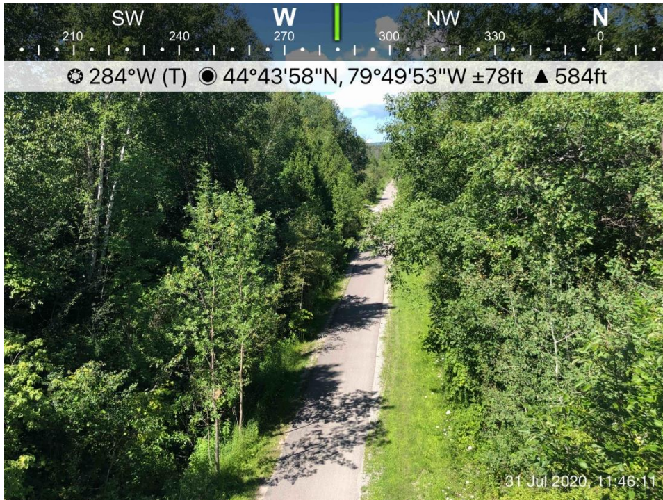
Photo 15: Photo taken facing west from the top of the bridge. July 31, 2020.
