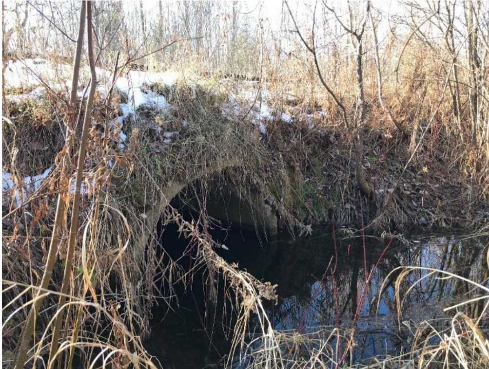
Image 32 Culvert under rail corridor; Area is disturbed, no potential
