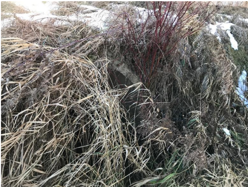
Image 19 Culvert under rail corridor; Area is disturbed, no potential
