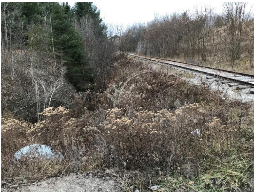
Image 51 Culvert under road; Area is disturbed, no potential
