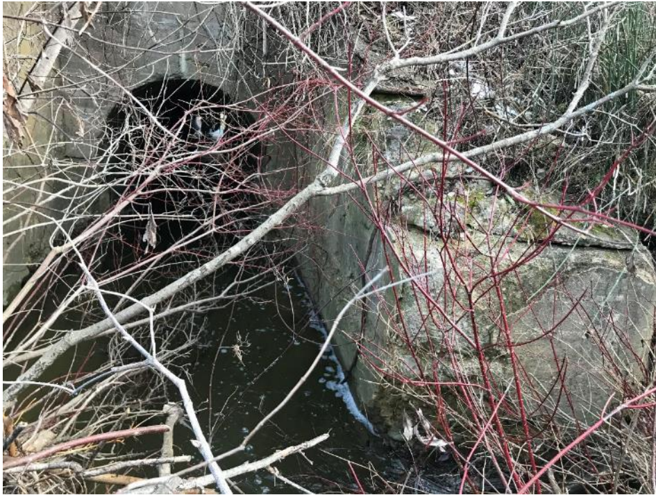
Image 6 Culvert under rail corridor; Channelized and culverted section of Warrington Creek is disturbed, no potential
