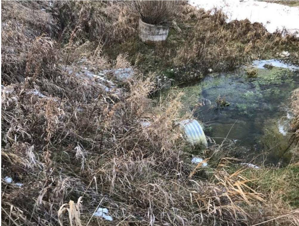
Image 18 Culvert under rail corridor; Area is disturbed, no potential
