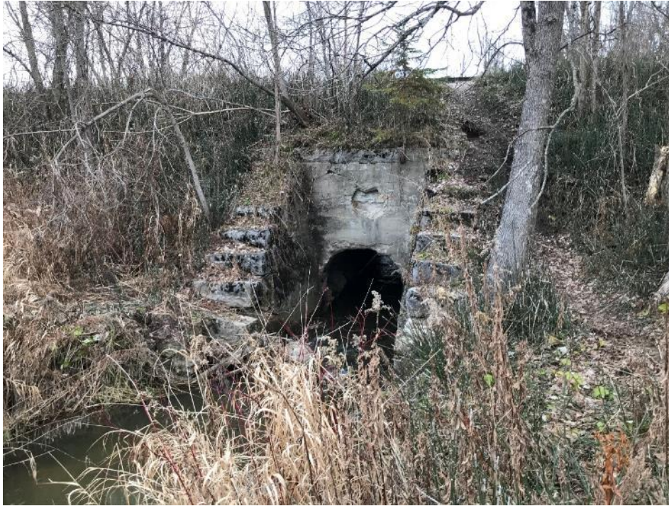
Image 50 Culvert under rail corridor; Area is disturbed, no potential
