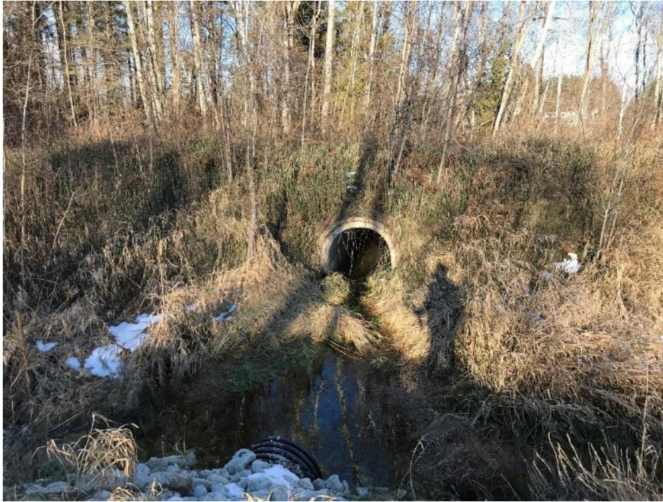
Image 24 Culvert under rail corridor; Area is disturbed, no potential
