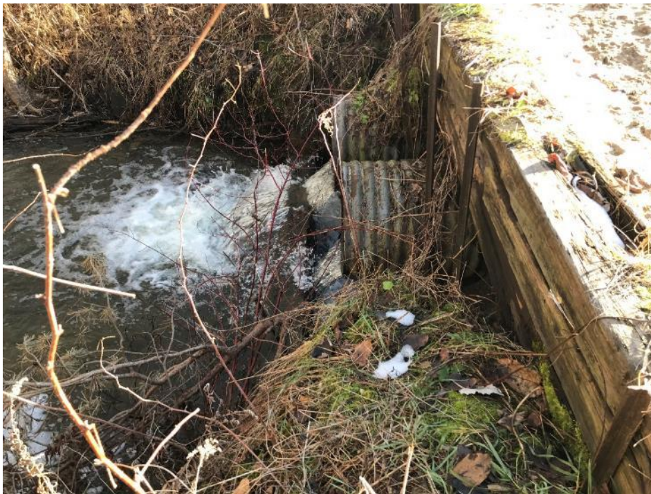
Image 33 Culvert under rail corridor; Area is disturbed, no potential
