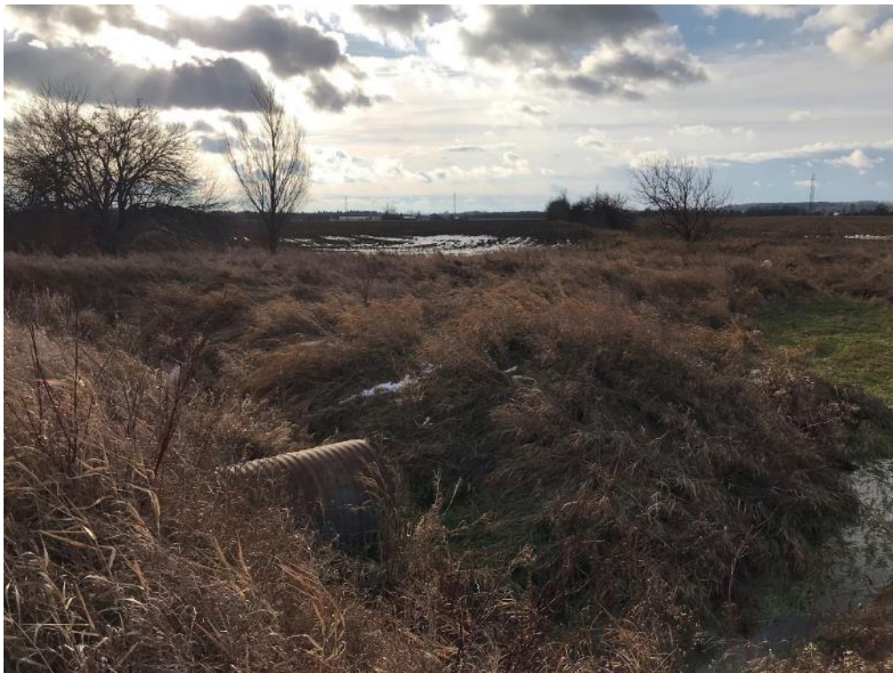
Image 15 Culvert under rail corridor; Area is disturbed, no potential
