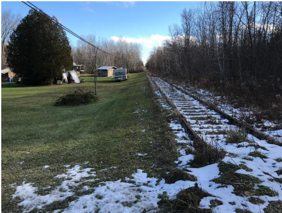
Image 31 View of rail corridor; Area beyond disturbed rail right-of-way requires Stage 2 survey
