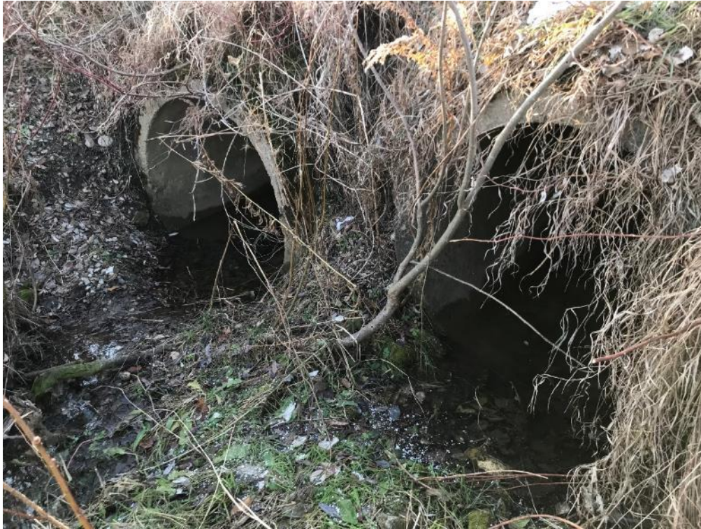
Image 14 Culvert under rail corridor; Area is disturbed, no potential
