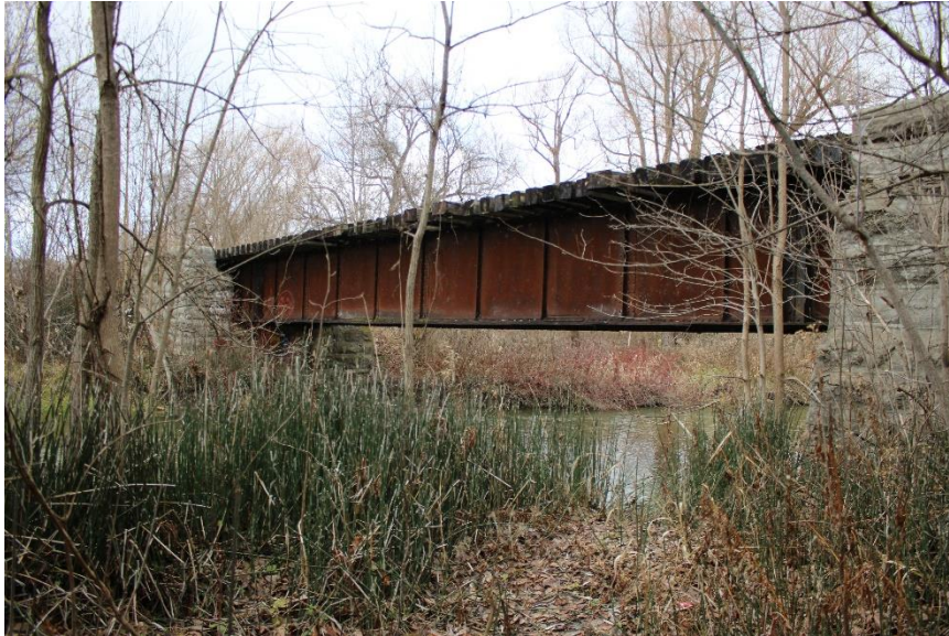
Plate 11: North elevation of the Pine River Bridge, looking southeast.
