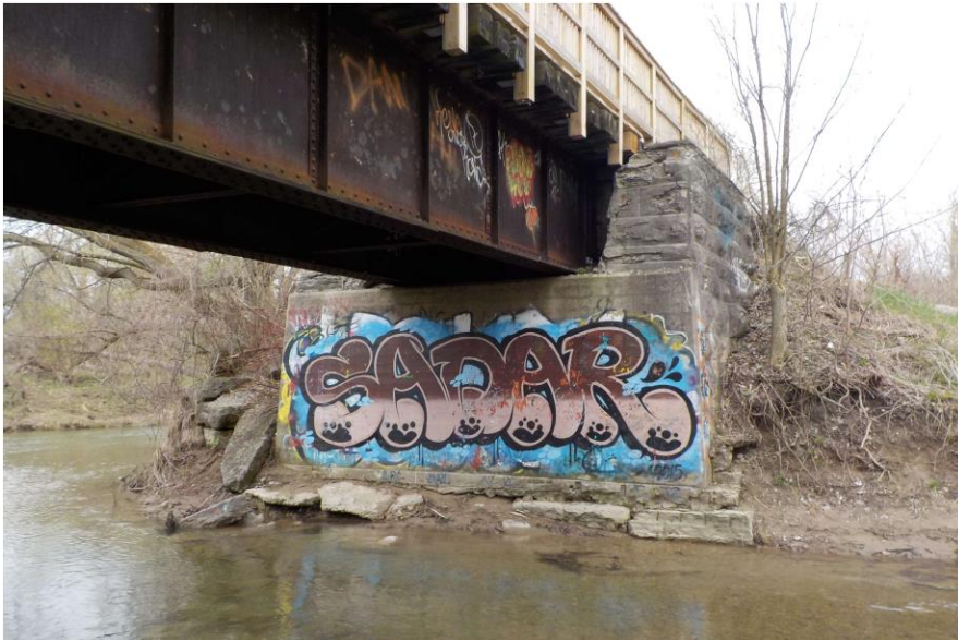
Plate 33: Barrie-Collingwood Railway Structure #2, Poplar Sideroad, Collingwood deck plate girder bridge (County of Simcoe n.d.)
