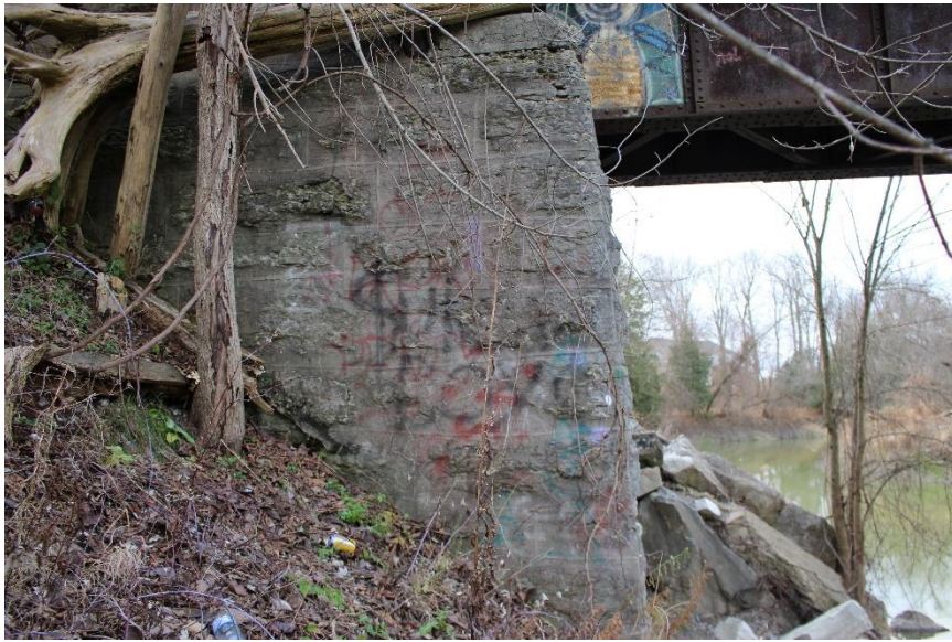
Plate 27: North elevation of the east abutment, looking south.
