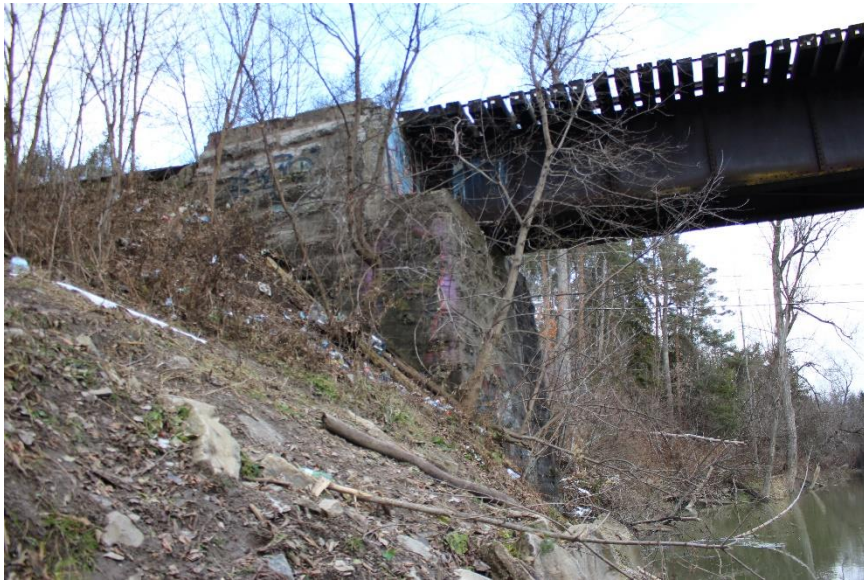
Plate 25: South elevation of the west abutments, looking north.
