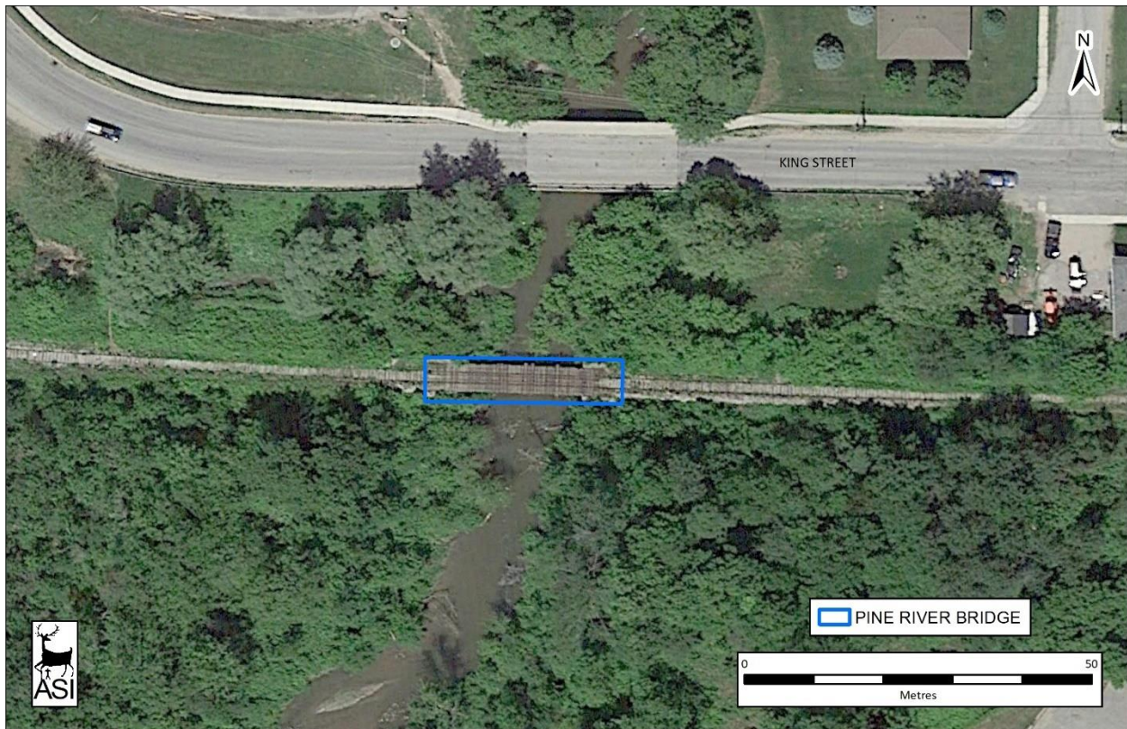
Figure 5: Satellite imagery depicting the location of the Pine River Bridge. Base Map: ESRI
