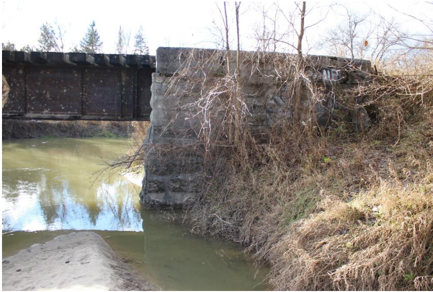
Plate 5: North elevation of the west abutments, looking south.
