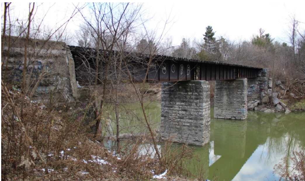
Figure 8: The south elevation of the Nottawasaga River Bridge (ASI 2021)
