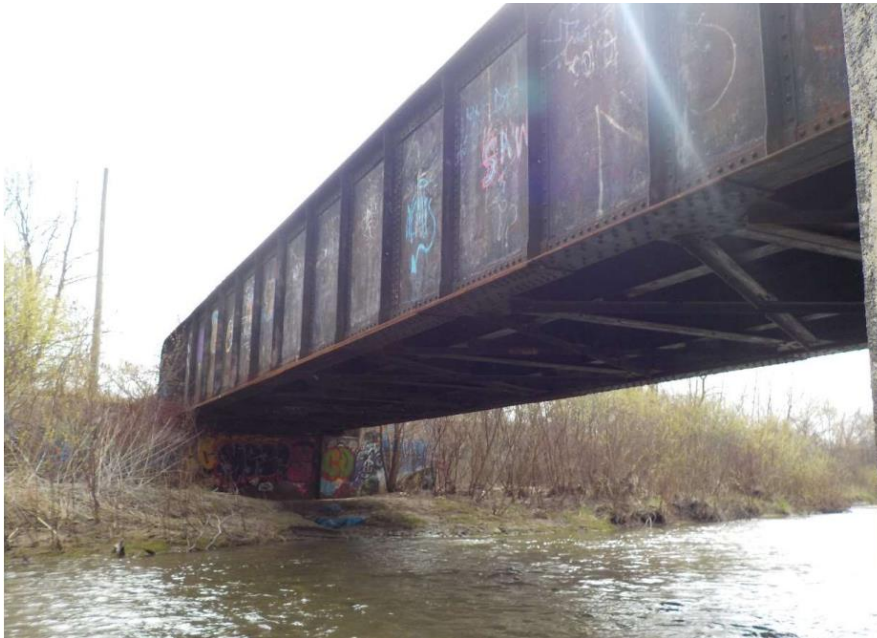
Plate 32: Barrie-Collingwood Railway Structure #1, Raglan Street, Collingwood though plate girder bridge (County of Simcoe n.d.)
