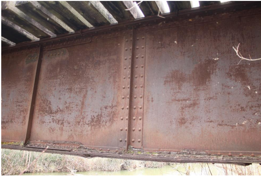
Plate 17: Detail of riveted plate girder on the north elevation.
