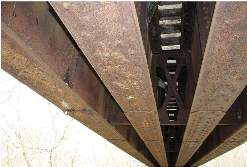
Plate 16: Superstructure soffit showing riveted connections and diaphragms between girders.
