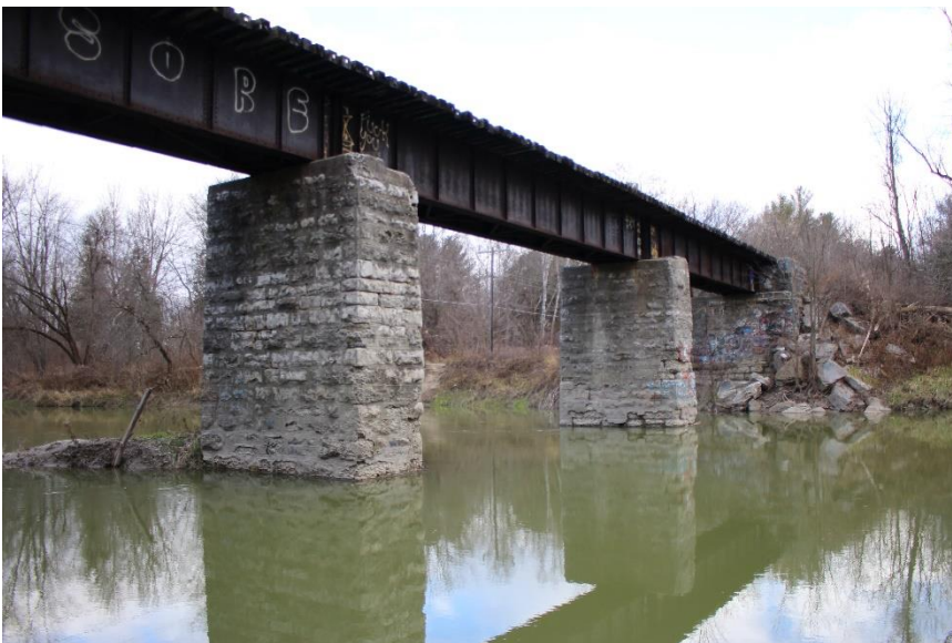
Plate 22: Oblique view of the stone masonry piers, looking northeast.
