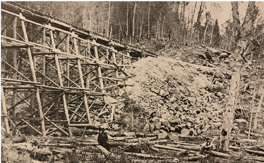
Figure 19: Trestle bridge infilling on the Ottawa, Arnprior, and Parry Sound Railway, in present day Algonquin Park, c. 1895 (Algonquin Park Archives item 125, in Mackay 1998:22)
