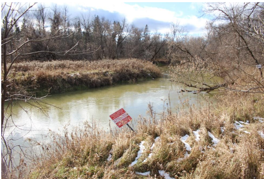
Plate 10: Mad Creek south of the subject bridge, with grasses and shrubs in the floodplain and mature trees at rear left, looking southwest.
