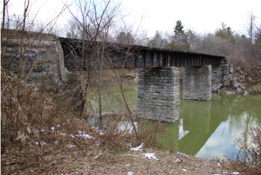
Plate 21: South elevation of the Nottawasaga River Bridge, looking northeast.
