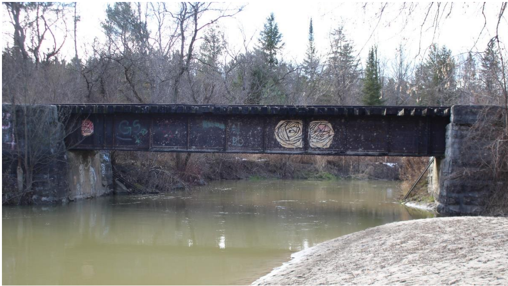
Figure 3: The north elevation of the Mad River Bridge (ASI 2021)
