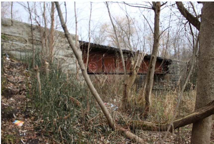
Plate 12: Oblique view of the south elevation, looking northeast.
