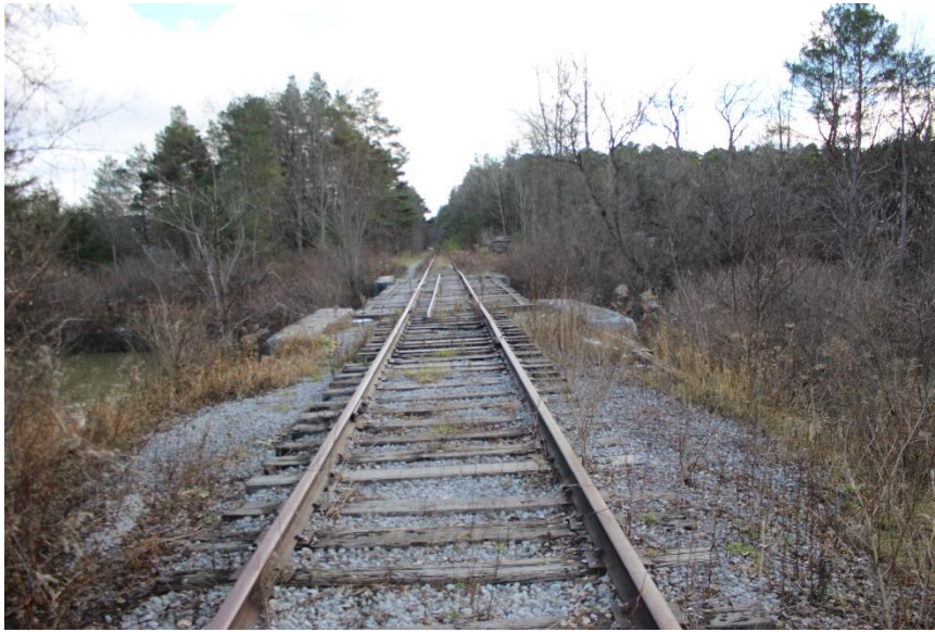
Plate 9: Rail corridor, looking east towards the subject bridge.
