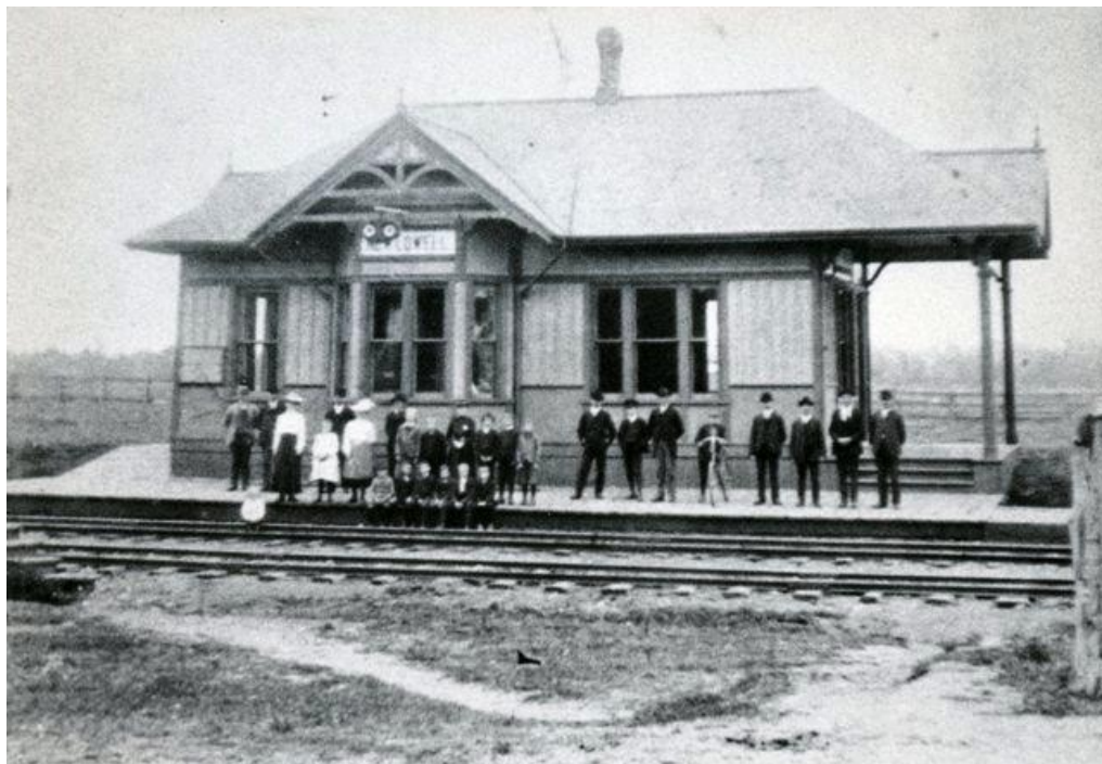
Figure 11: Photograph of New Lowell Station on the former OS&HU, unknown date (Cooper 2014)
