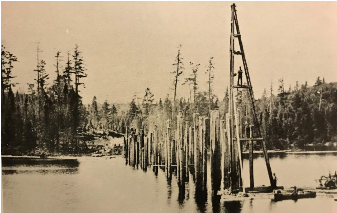
Figure 20: Trestle bridge piling being driven into a lake for the on the Ottawa, Arnprior, and Parry Sound Railway, in present day Algonquin Park, 1896 (Algonquin Park Archives item 146, in MacKay 1998:25)
