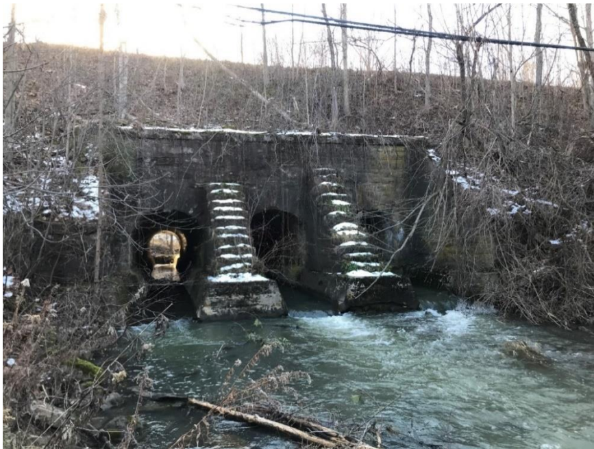
Plate 8: View of the New Lowell stone arch culvert, looking west.
