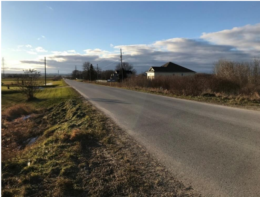
Plate 5: Concession Road 7 Sunnidale, looking west.
