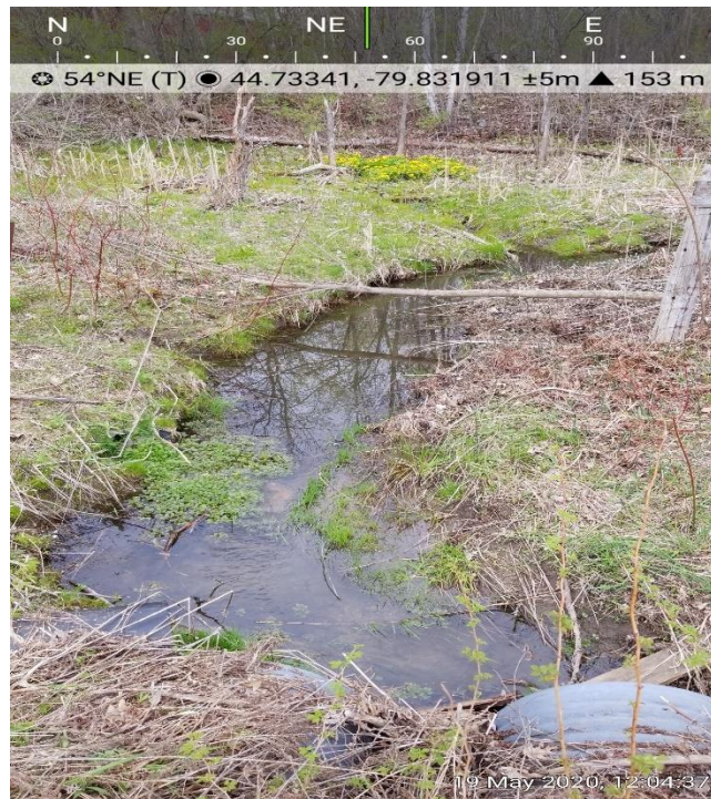
Photo 2: Looking upstream from culvert inlet.
