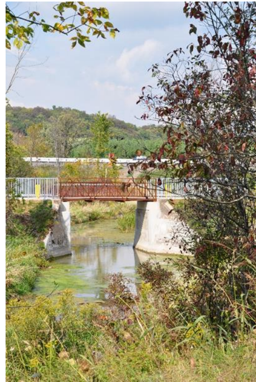
Figure 24: Left – New trail bridge using former railway abutments, K&P Trail Kingston, ON. Right – Trail bridge retrofit onto former railway structure, Caledon Trailway Caledon East ON (source WSP)
